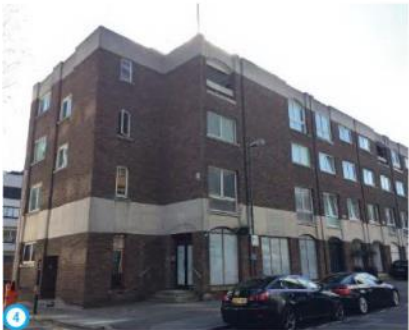
4 Building B from Blandford Street
